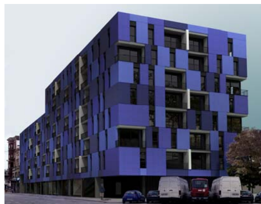
LOCALS ADEQUATS PER A INVERSORS
