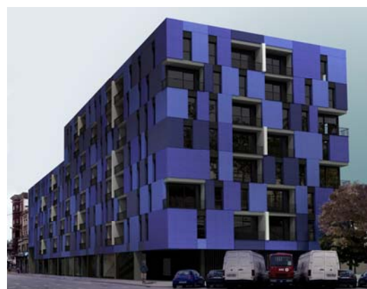
LOCALS ADEQUATS PER A INVERSORS
