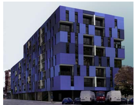
LOCALS ADEQUATS PER A INVERSORS
